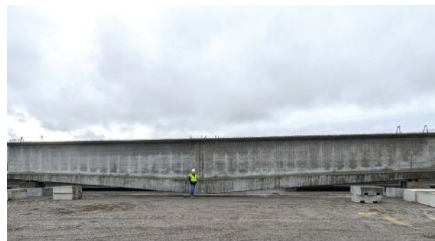
Lightweight concrete haunched pier girder segment for the North Spokane Corridor Bridge over the Spokane River. Photo credit: Jordan Pelphrey.
