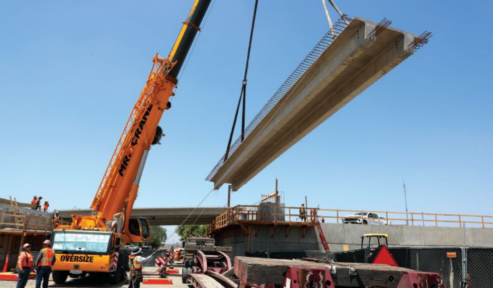
Setting of a prestressed concrete Northeast Extreme Tee (NEXT) girder at the 3rd Street overcrossing. The shallow 28-in.-deep NEXT girder is used to provide the 15-ft minimum vertical clearance. Photo: Dany Schimpf Photography.
