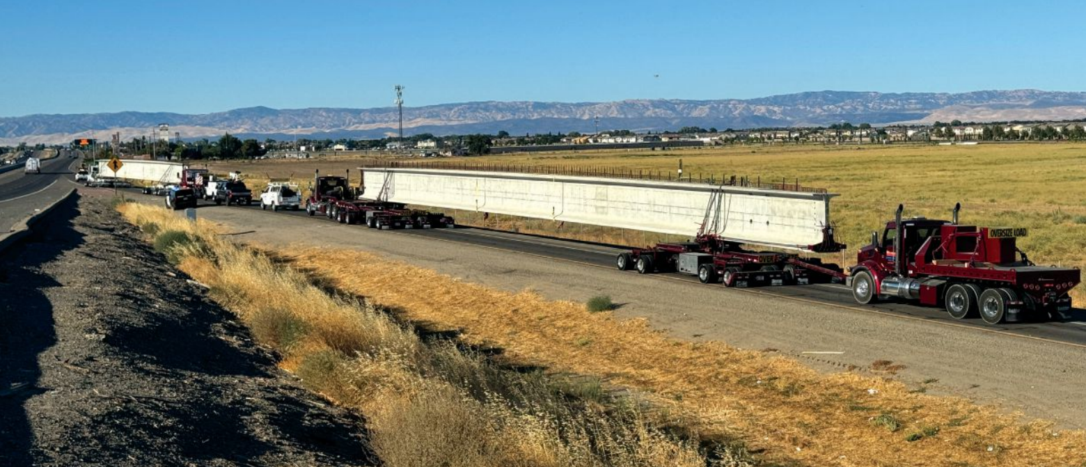
The California WF84 girders are transported to the site using specialized hauling equipment to accommodate the weight and length of the large girders. Photo: Dany Schimpf Photography.
