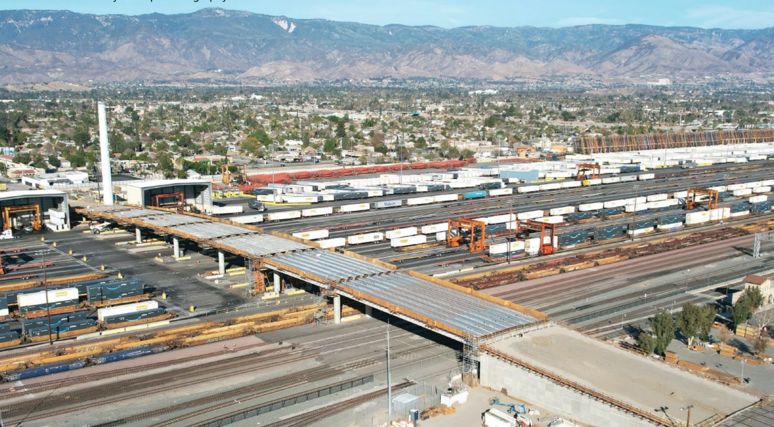
The new seven-span Mount Vernon Viaduct bridge and the one-span 3rd Street crossing use precast, prestressed concrete girders. Photo: Dany Schimpf Photography.
