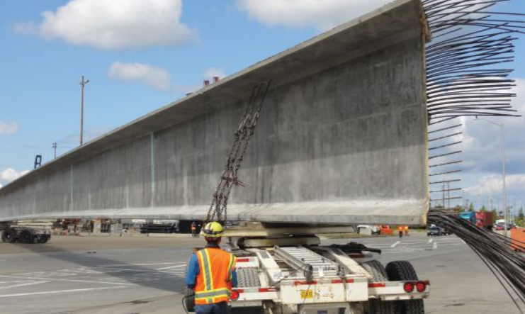
The longest prestressed concrete girders in Washington state are installed on southbound Interstate 5 Puyallup River Bridge in Tacoma. These girders measure 223 ft in length and almost 9 ft in height, and each weighs more than 246,500 lb.
