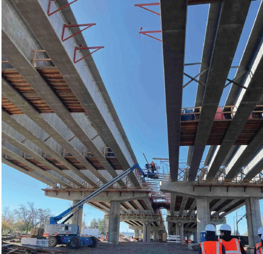
View from beneath the erected WF83G pretensioned concrete girders. Photo: Kuney Construction.
