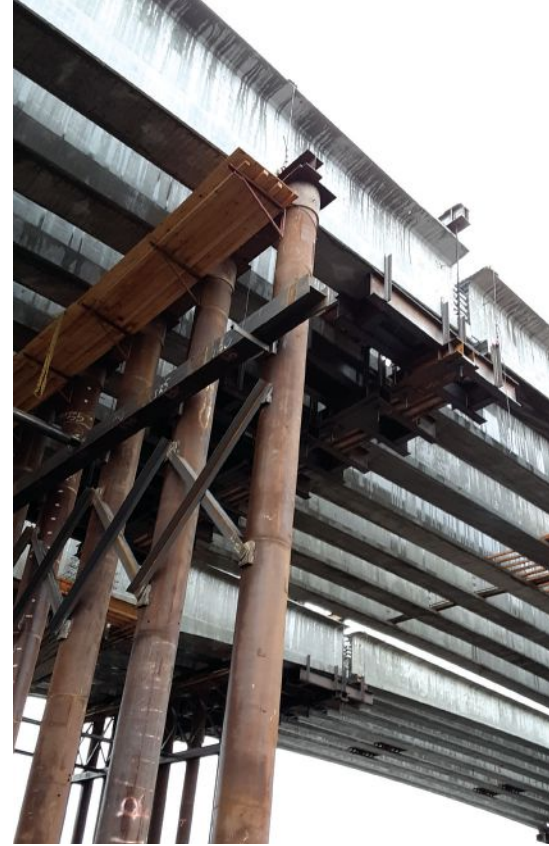
Prestressed concrete drop-in segments suspended from the haunched girder segments whose ends are temporarily supported by falsework before post-tensioning is installed. Photo: Kris Brown.
