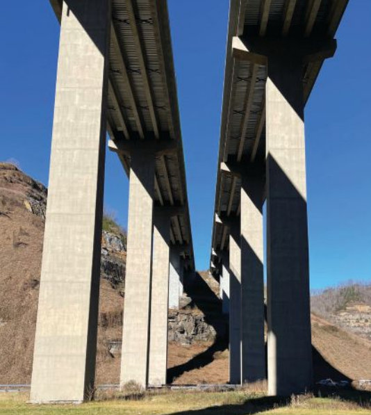
Part of the Corridor Q project, this bridge carrying U.S. Route 460 over Marrowbone Creek and Kentucky Route 195 features twin nine-span precast concrete I-beam structures with 180-ft-tall piers. The structure is supported on tapered, hollow piers. Photo: Palmer Engineering.
