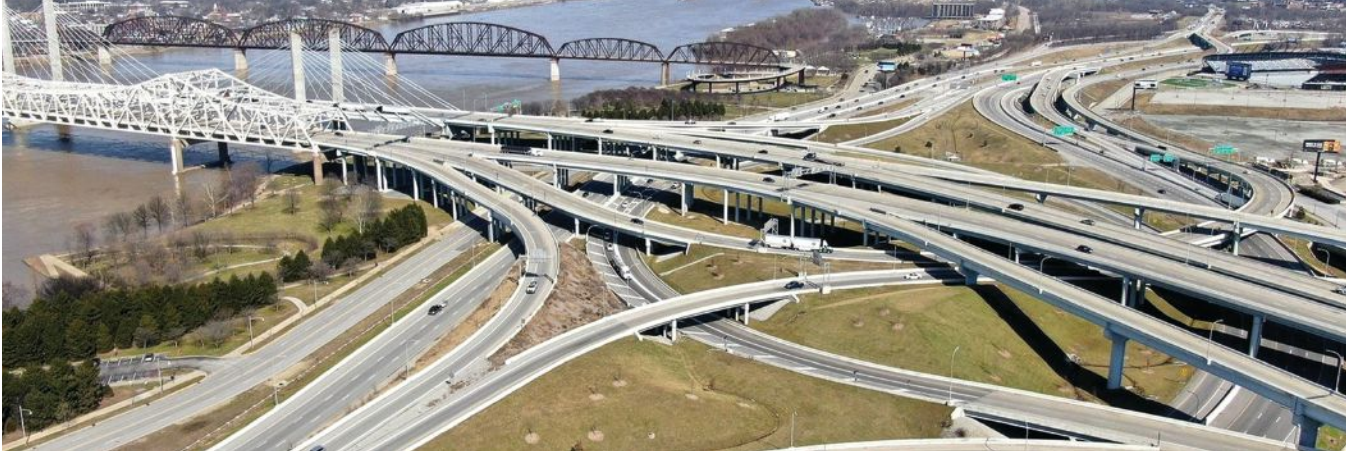
The Kennedy Interchange—also known as “Spaghetti junction”—is the confluence of three interstates and intertwines with local access roads between downtown Louisville, Ky., and the Ohio River. Palmer Engineering was part of the project team that designed the reconstruction of the interchange. Photo: Palmer Engineering.
