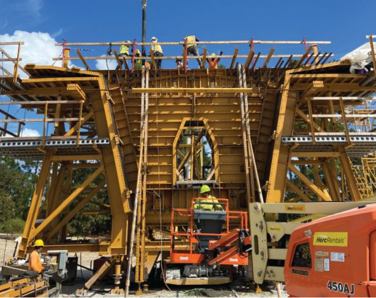
Casting of a pier segment at the precast concrete manufacturer's facility for the Interstate 26 project.
