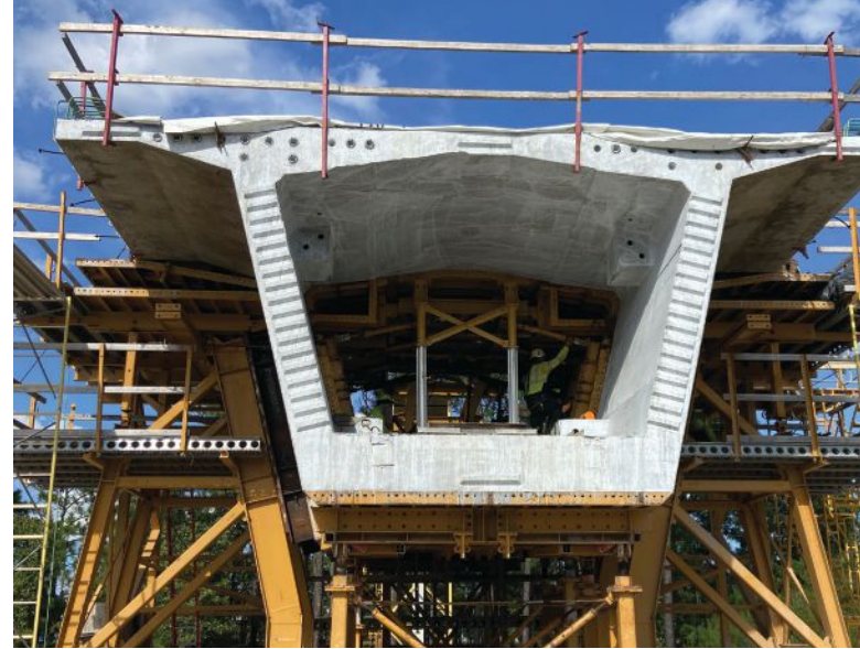
A variable-depth typical precast concrete segment for the Laurel Fork project is in position for the next segment to be match cast against it in the adjacent casting cell.
