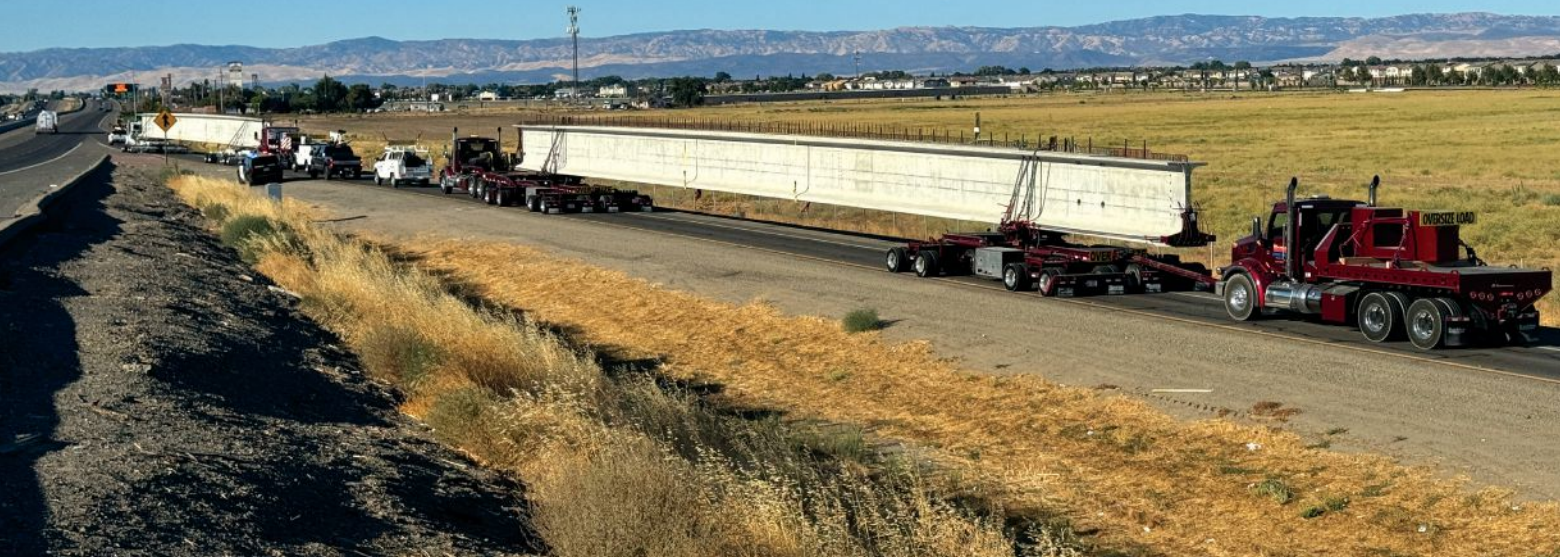
The California WF84 girders are transported to the site using specialized hauling equipment to accommodate the weight and length of the large girders. Photo: Dany Schimpf Photography.
