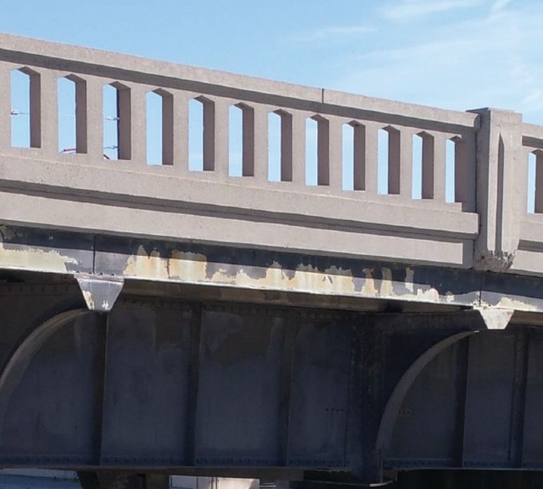
Detail of an original steel corbel on the old bridge at the sidewalk (left) and a rendering of the precast concrete corbel detail for the new viaduct (right). Photo (left): San Bernadino County Transit Authority. Figure (right): COWI.
