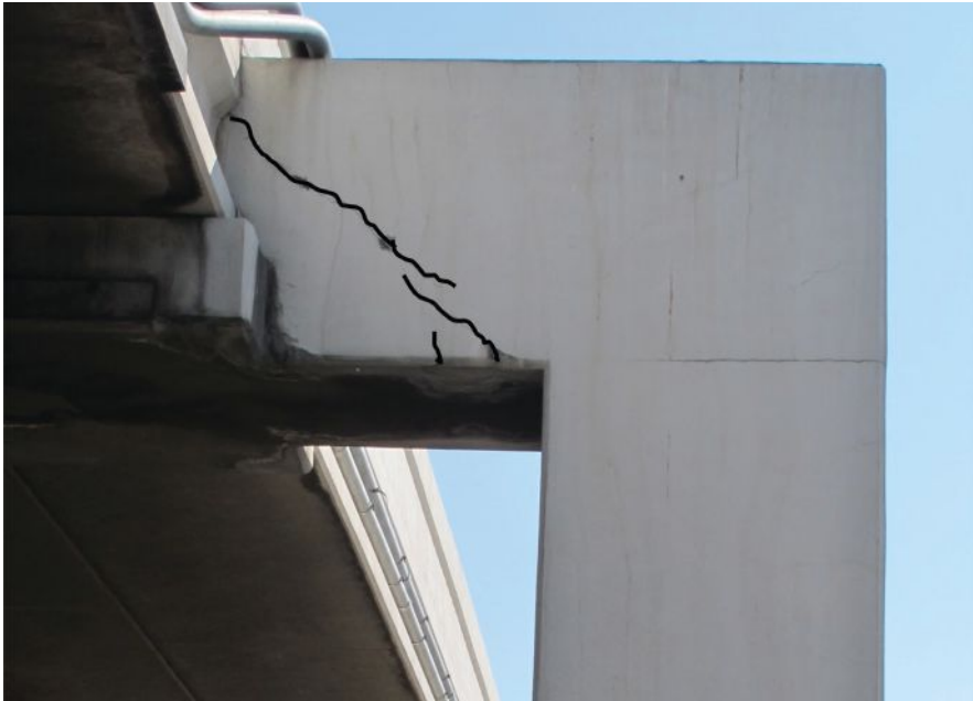
Figure 4. Straddle bent with an inverted-tee cross section has shear cracks. Cracks have been enhanced. Source: Adapted from Larson et al. 7
