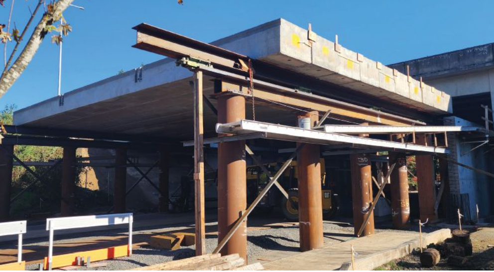
First group of prestressed concrete slabs are ready for lateral translation. Photo: David Evans and Associates Inc.
