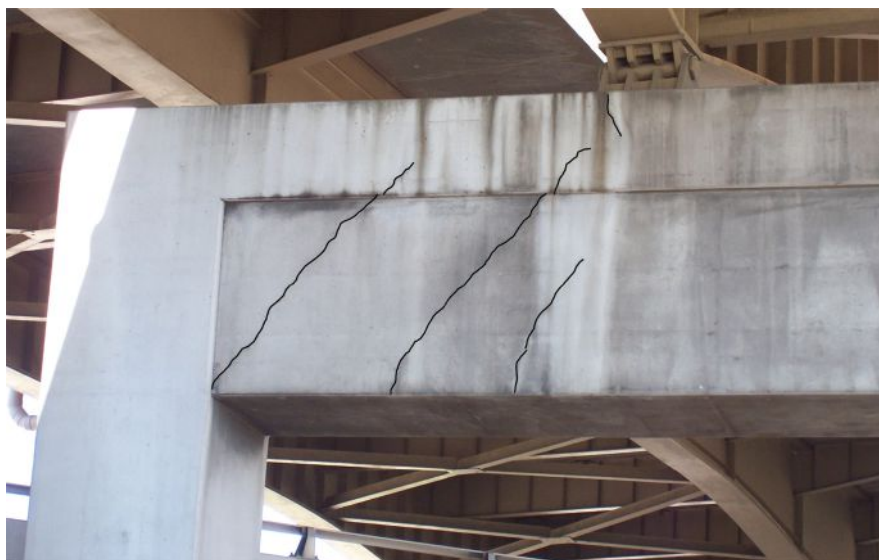
Figure 3. Multicolumn bent with both shear and shear-flexure cracks. Cracks have been enhanced. Source: Adapted from Birrcher et al. 6
