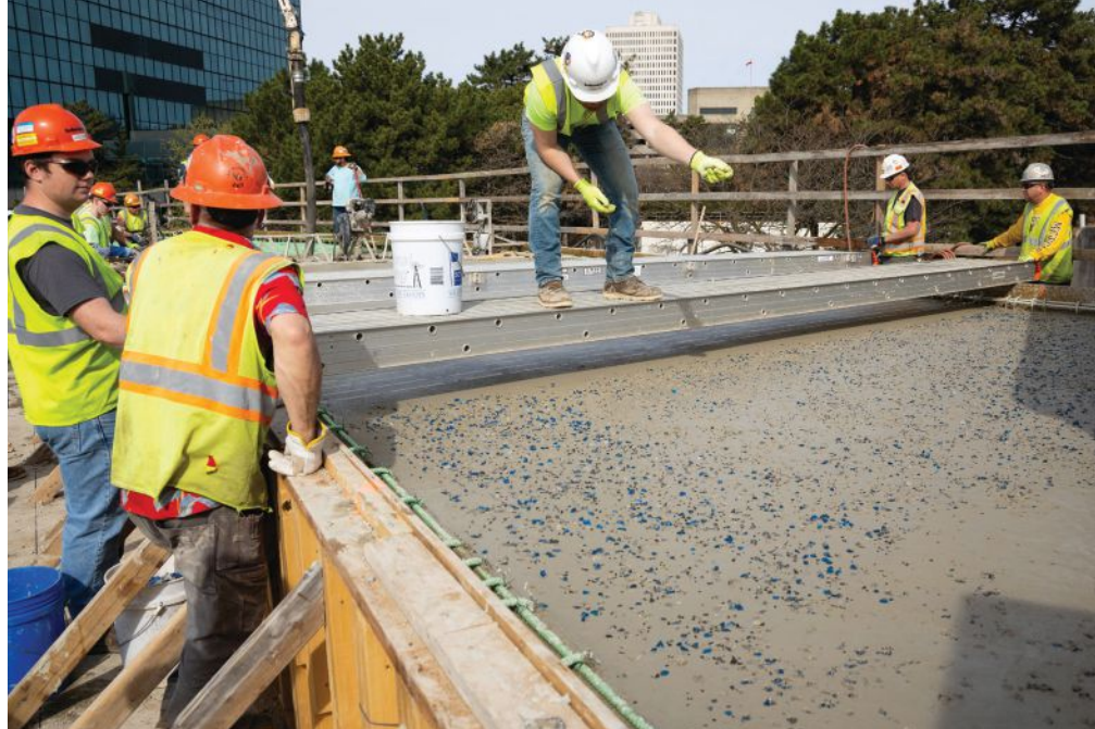
Workers perform the first step in creating a glass-seeding finish by applying a mix of tumbled glass (blue, white, and gray colors) on the fresh concrete surface, just after it was finished. The glass seeding enhances the bridge aesthetics and recalls Toledo's history as the Glass City. Photo: Colliers Engineering & Design.
