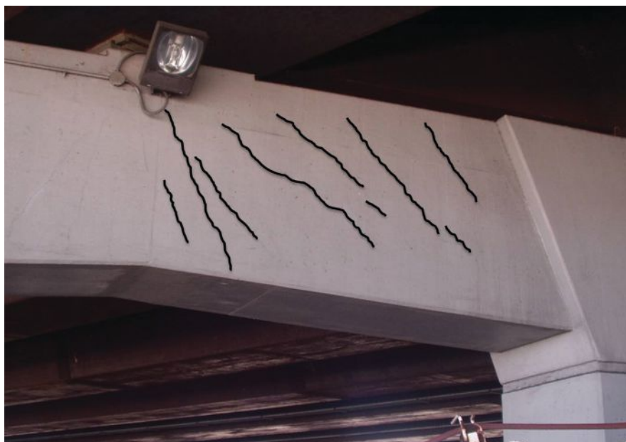
Figure 3. Multicolumn bent with both shear and shear-flexure cracks. Cracks have been enhanced. Source: Adapted from Birrcher et al. 6
