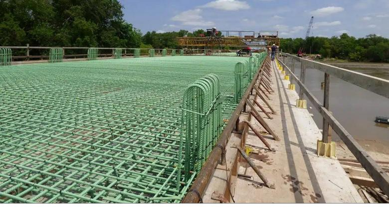
Epoxy-coated reinforcing steel provides long-term corrosion protection in bridge applications, especially in areas exposed to deicing salts and moisture such as the driving surface of the Mount Hope Bridge (shown here), which spans the Arkansas River in Kansas.
