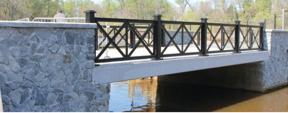
General elevation view of new bridge taken from the pond side, looking southwest. Decorative stone facing runs along the existing parapets on the bridge approaches and extends down the outside face of the abutments and wingwalls.
