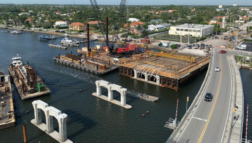
Spans 1 and 2 before concrete placement. Photo: Florida Department of Transportation.
