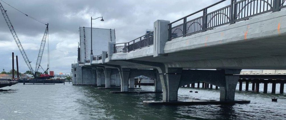
The completed east approach spans with the drawbridge visible in the background. Photo: H&H.
