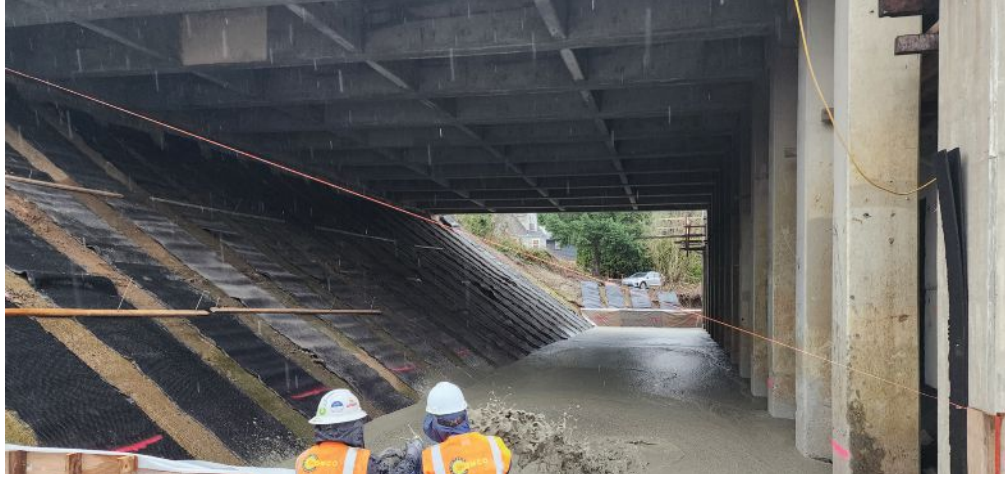
Low-density cellular concrete (LDCC) backfill is placed behind the new abutments. LDCC backfill was used to achieve a near net-zero overburden pressure on the excavated surface. Photo: David Evans and Associates Inc.
