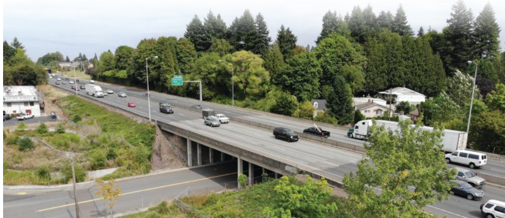
Only a single 56-hour closure was required for replacement of the Interstate 5 bridge over SW 26th Avenue in Portland, Ore. Photo: David Evans and Associates Inc.
