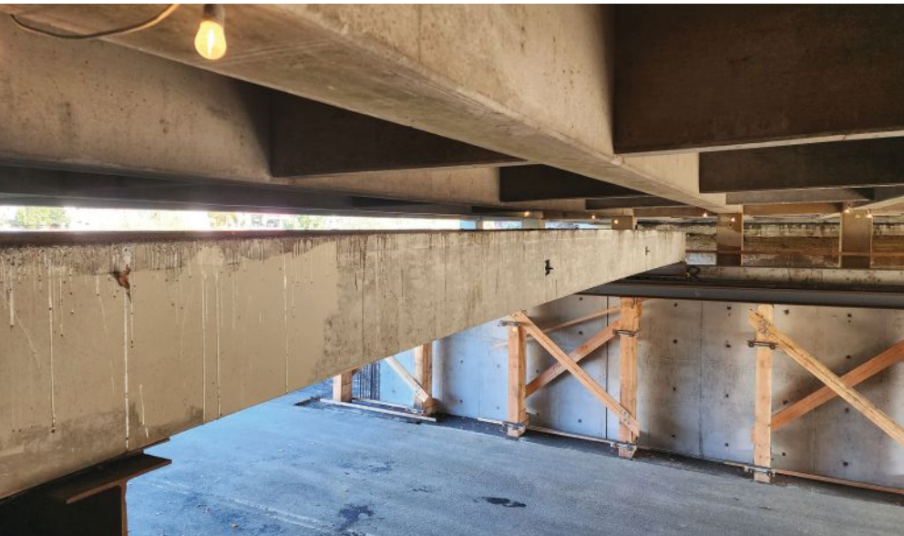
Translation of the first stage of precast concrete slabs under the existing bridge. Photo: David Evans and Associates, Inc.
