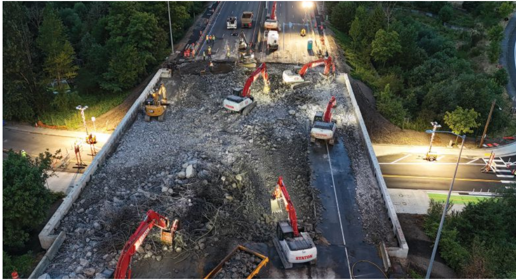
Demolition of the existing superstructure during the weekend closure. The debris was used as roadway fill, which kept the material out of the landfill. Photo: Oregon Department of Transportation.
