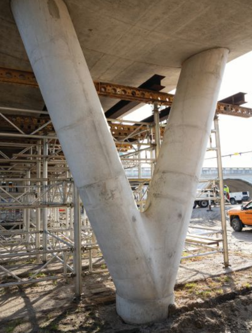
Elevation view of one of the finished V-shaped piers showing the architectural form, including the smooth fillet area between the column legs. Photo: Colliers Engineering & Design.
