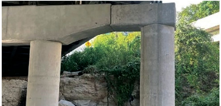
Figure 6. Example of bridge widening where forces are transferred across newly created interfaces. Photo: Concrete Bridge Engineering Institute.
