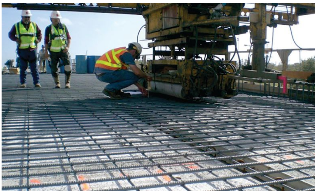
Figure 1. After the deck has been thoroughly wetted and prepared, workers use a screed to level cast-in-place concrete on top of a precast concrete panel. 3
