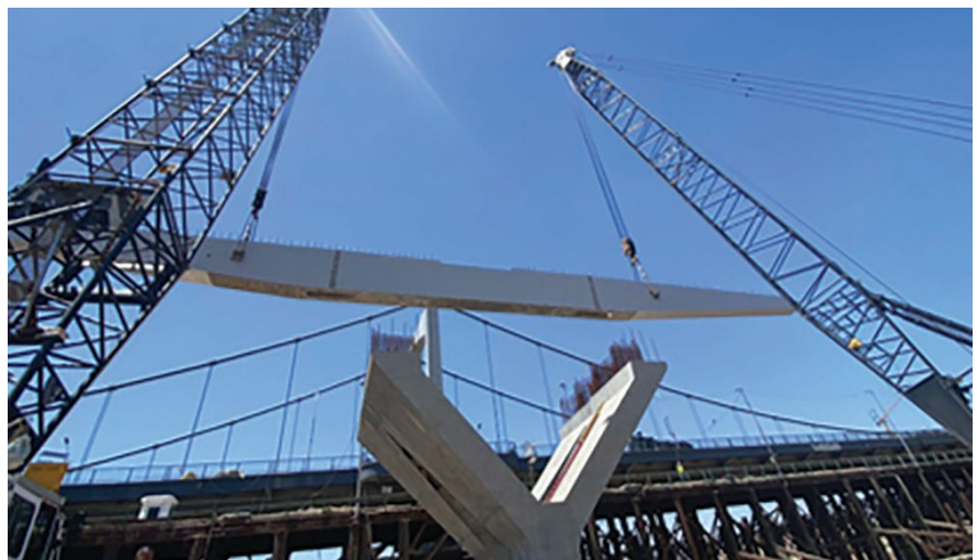
Figure 7. Installation of the first and second precast concrete U-shaped haunch girders.
