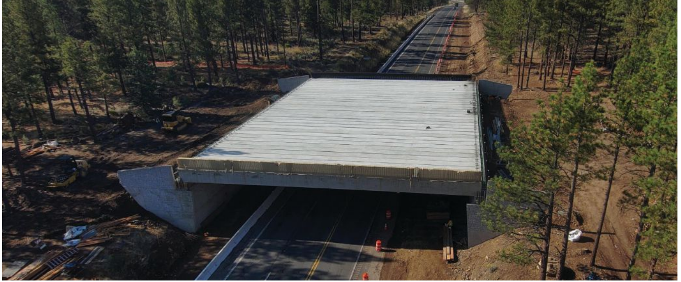
The Grass Lake Wildlife Overcrossing is composed of precast, prestressed concrete box girders. The girders, which each contain thirty-five 0.6-in.-diameter strands, were designed to achieve an initial concrete compressive strength of 7000 psi and a final concrete compressive strength of 8000 psi. Photo: California Department of Transportation.
