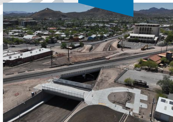
Photo: Downtown Links Constructors.
