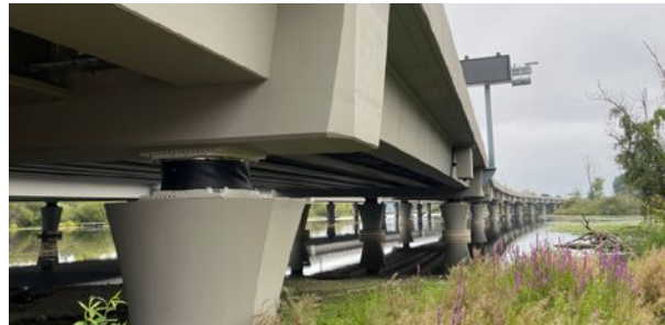
Photos: Graham Contracting and TYLin.
