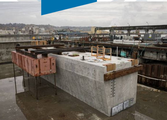
Photo: Manson Construction.
