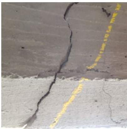
Figure 3. A crack with vertical offset at web soffit that was observed during a routine biennial inspection of Mosier Bridge no. 07626A in 2013 (left); flexural bar cutoff location superimposed over the interior girder of the bridge (right). The bridge was immediately shored pending analysis and strengthening. Photo: Oregon Department of Transportation.
