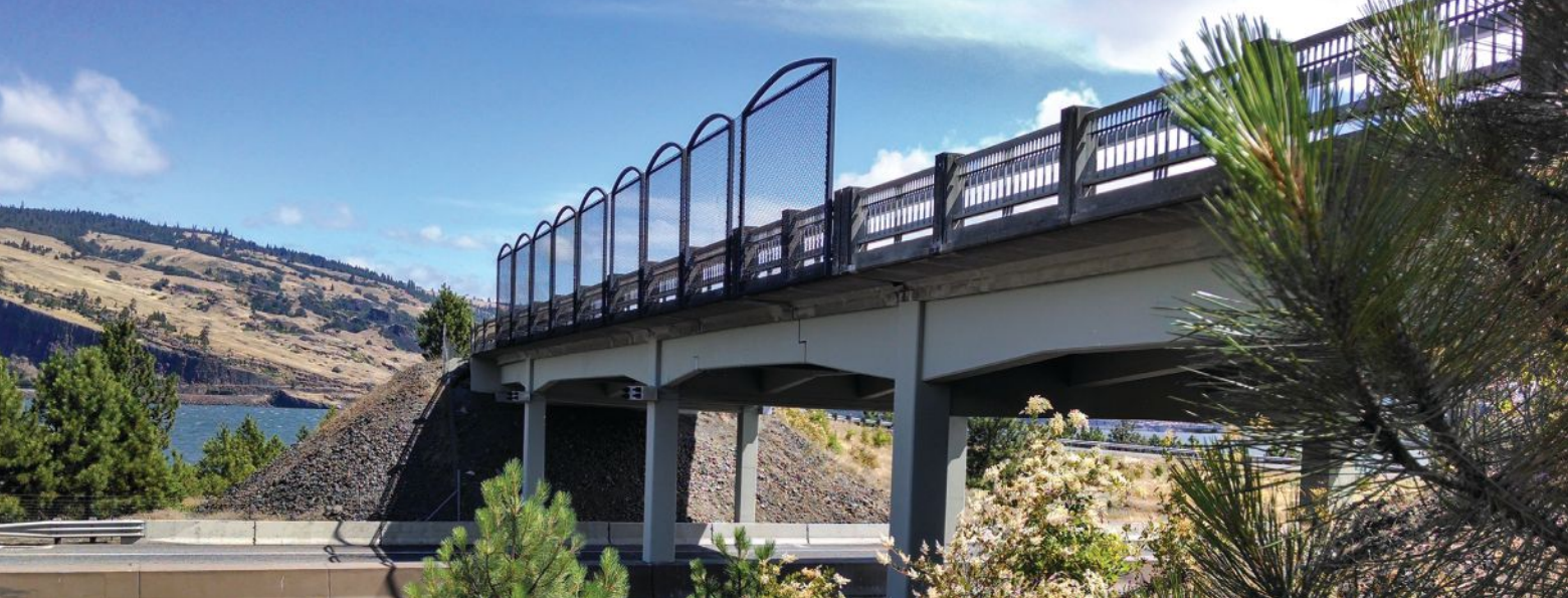
Figure 6. Photo of the completed Mosier Bridge no. 07626A, a two-lane, three-span continuous reinforced concrete deck girder bridge that has four girder lines with girders spaced at 8 ft 8 in. The bridge was strengthened in the field, with near-surface-mounted titanium alloy bars proving to be the most practical strengthening option given the geometry of the haunch at the critical section. Photo: W. George.
