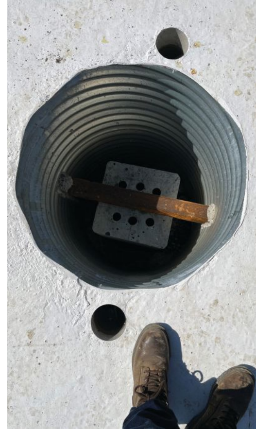
The precast concrete abutments were built with eight 30-in.-diameter full-depth voids, which were created by casting corrugated metal pipes. These voids were essential for proper connection between the precast concrete piles and abutment sections.
