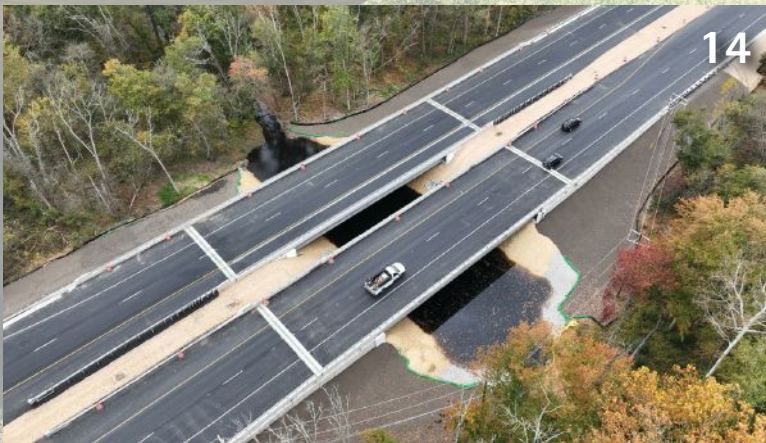
Photo: Delaware Department of Transportation.
