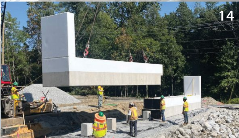
Photo: Delaware Department of Transportation.
