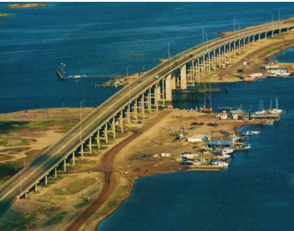
Figure 1. JFK Memorial Causeway in Texas is recognized as the first precast, post-tensioned concrete segmental bridge built in the United States. Built in 1973, the structure connects Corpus Christi to North Padre Island. All Figures and Photos: American Segmental Bridge Institute.
