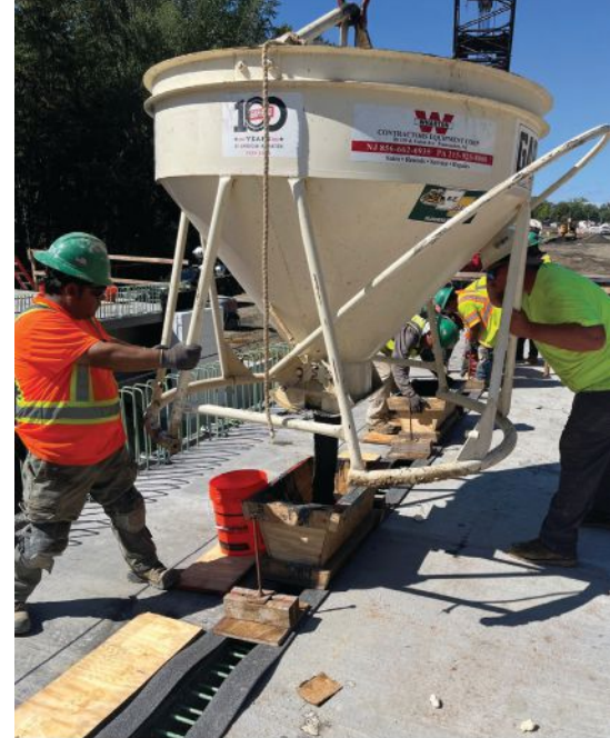
Workers place ultra-high-performance concrete (UHPC) from a concrete hopper into a longitudinal joint between adjacent decked bulb-tee beams. After the UHPC is placed, the joint is top formed and a pressure head system is created.
