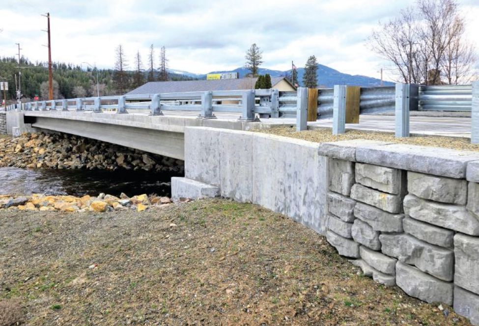
This structure over the Little Pend Oreille River has a 45-degree skew. Nicholls Kovich Engineering provided structural design, hydraulic analysis, and construction management.
