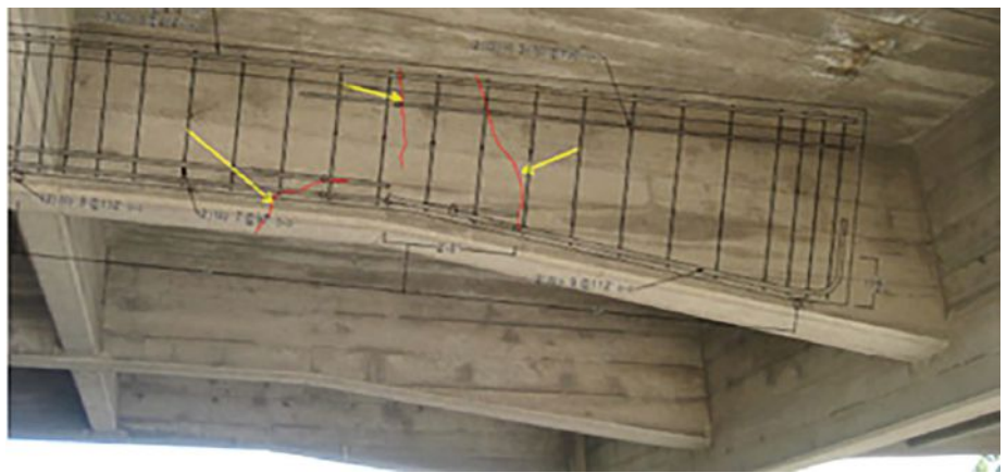
Figure 3. A crack with vertical offset at web soffit that was observed during a routine biennial inspection of Mosier Bridge no. 07626A in 2013 (left); flexural bar cutoff location superimposed over the interior girder of the bridge (right). The bridge was immediately shored pending analysis and strengthening. Photo: Oregon Department of Transportation.
