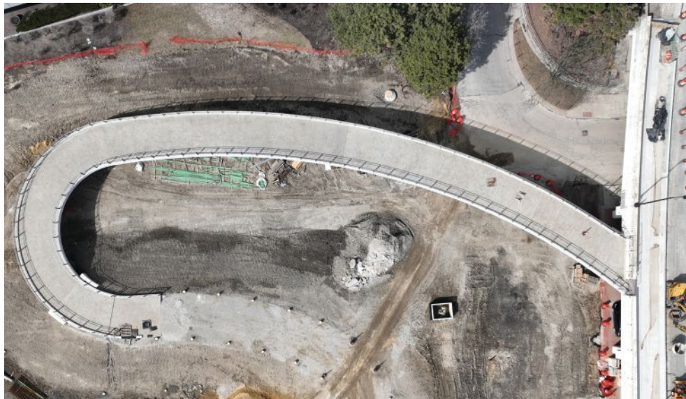
Figure 1. The Wood-Armer method was used for the design of the Bend Bridge, a curved, multispan, continuous, reinforced concrete slab bridge. Photo: Metroparks Toledo.
