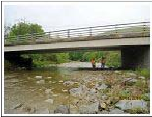
Figure 5 New York Pilot Bridge
