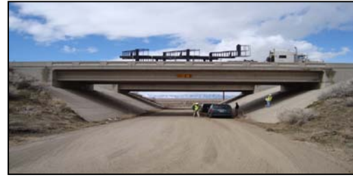
Figure 2 Utah Pilot Bridge
