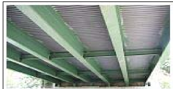
Figure 4 New Jersey Pilot Bridge
