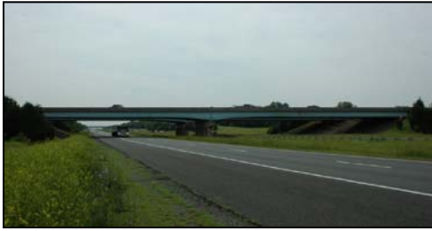
Figure 1 Virginia Pilot Bridge
